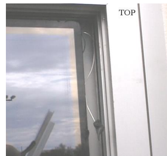
Do Install Glass With Tube in Upper Corner and Pointing Down
